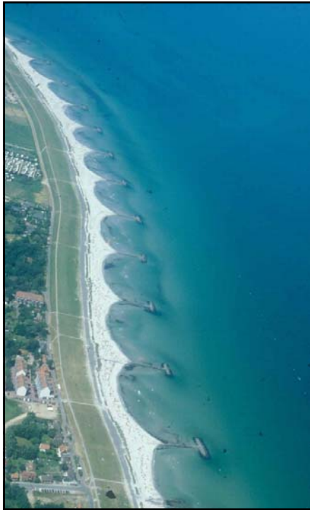
Coastal defence structures in the southern part of Kiel Bay (Baltic Sea). Dyke with T-groyne elements and additional beach nourishments.
