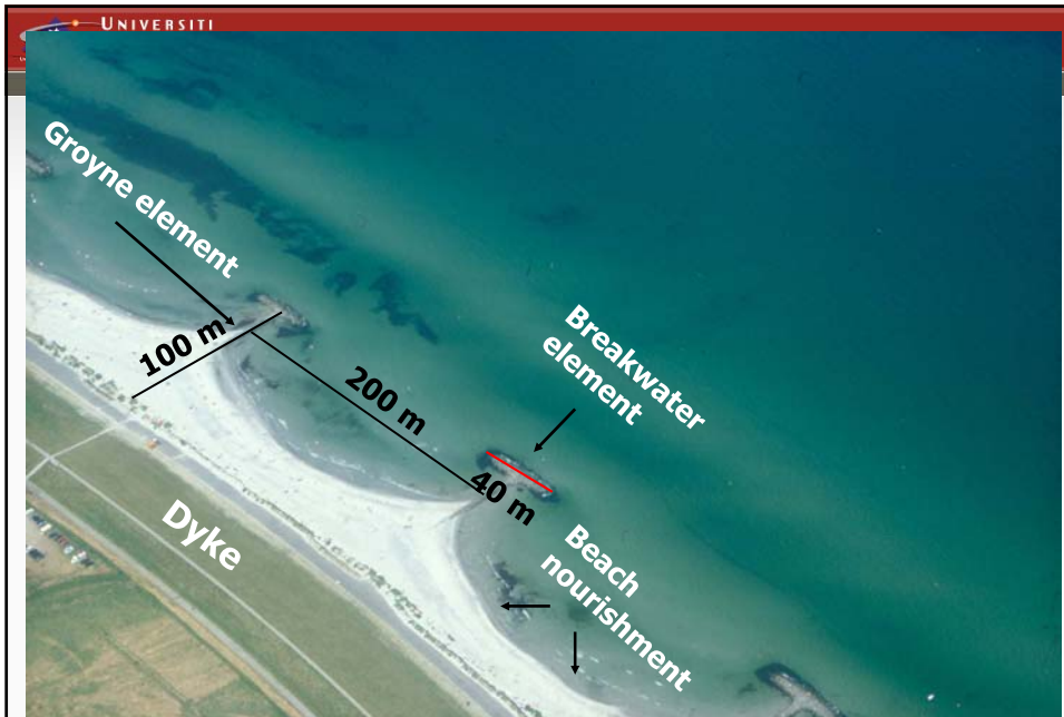
Coastal defence structures in the southern part of Kiel Bay, Probstei area (Baltic Sea). Dyke with T-groyne elements and additional beach nourishments.
